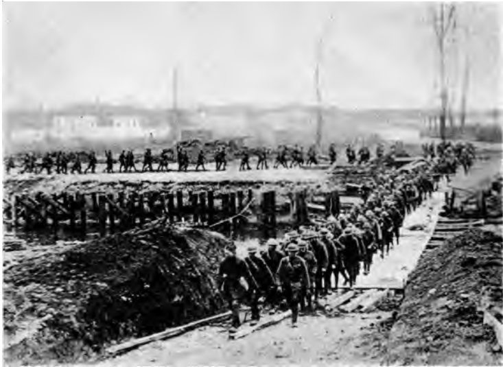
Men of Company A, 316th Engineers, marching over completed pontoon bridge constructed over River Scheldt. Taken on outskirts of Audenarde, Belgium.
